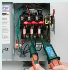
Conduct a 3-Phase Sequence Test
